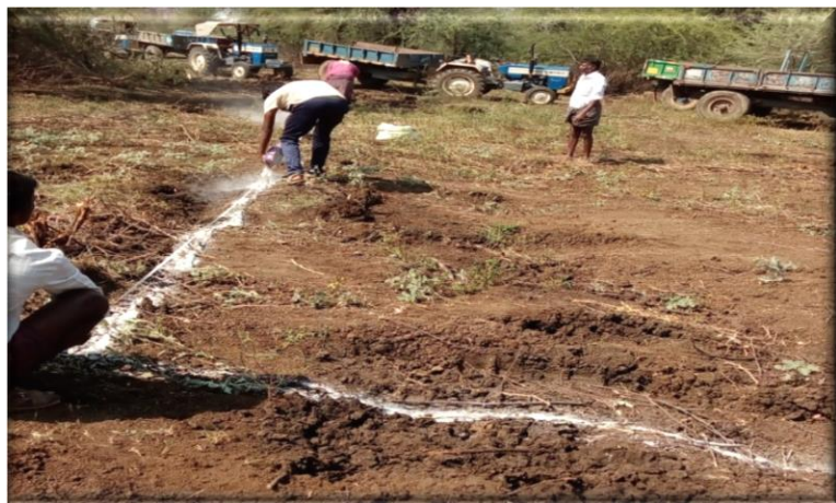
Marking out the tank
