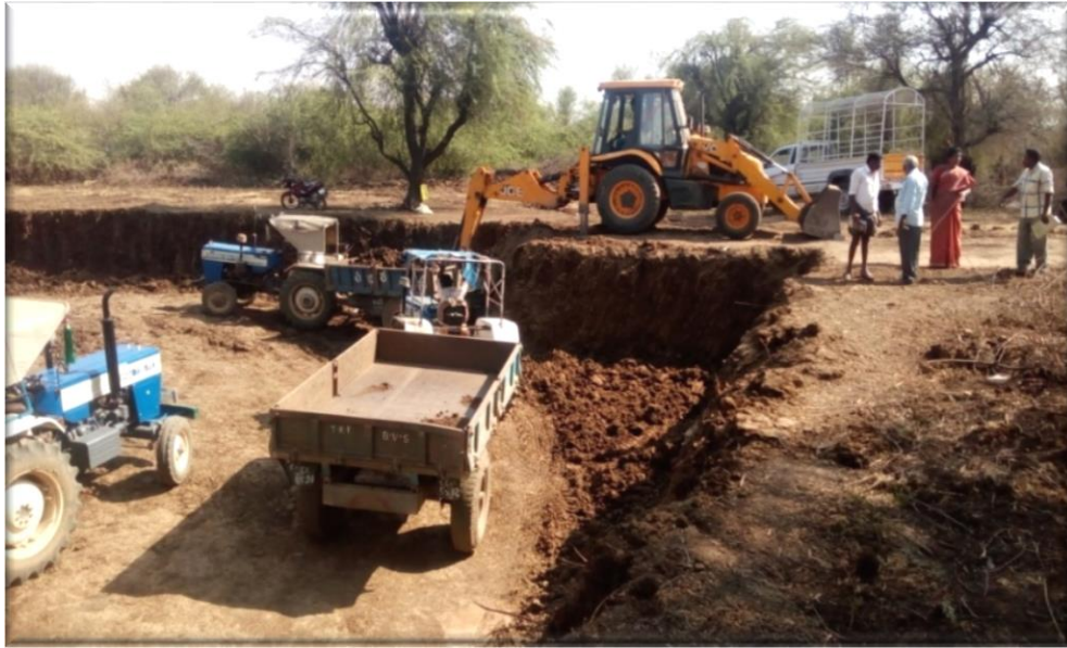
Working on the desilting
