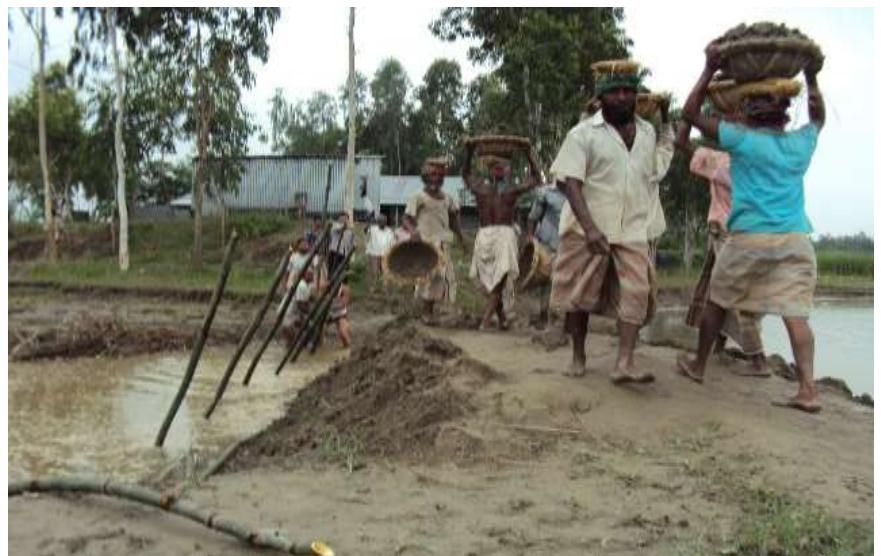
Community workers at the JRDP creating high ground by moving sand one basketful at a time. Photo courtesy Symbiosis Bangladesh.
