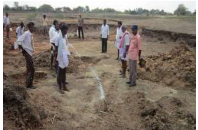
Marking out tank excavation at Buchepalli
