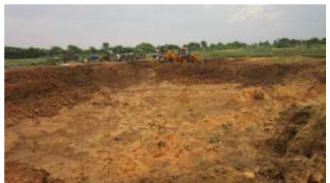
The end result - ready for the rain.
